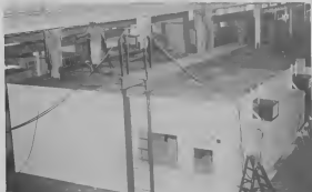
THIS NOISE-EXCLUDING office for Powerhouse No. 1 operators was designed by M. G. Murray, M. Croes and L. J. A. Halley. E OFICINA aki pa exclui zonida den Powerhouse No. 1 pa operadornan ta disenjá pa M. G. Murray, M. Croes y L. J. A. Halley.
